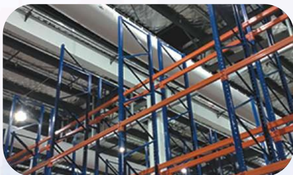
Xiaoyaoyao Group (Jinan) Medicine Cooling Warehouse
