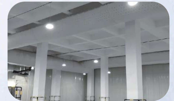
China Supply and Marketing International Livestock (Taixing) Cold Chain Logistics Park
