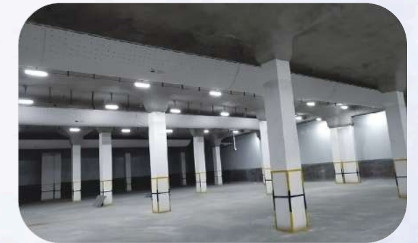
Cold Storage of Agricultural Product E-commerce Logistics Park in Northern Guiyang
